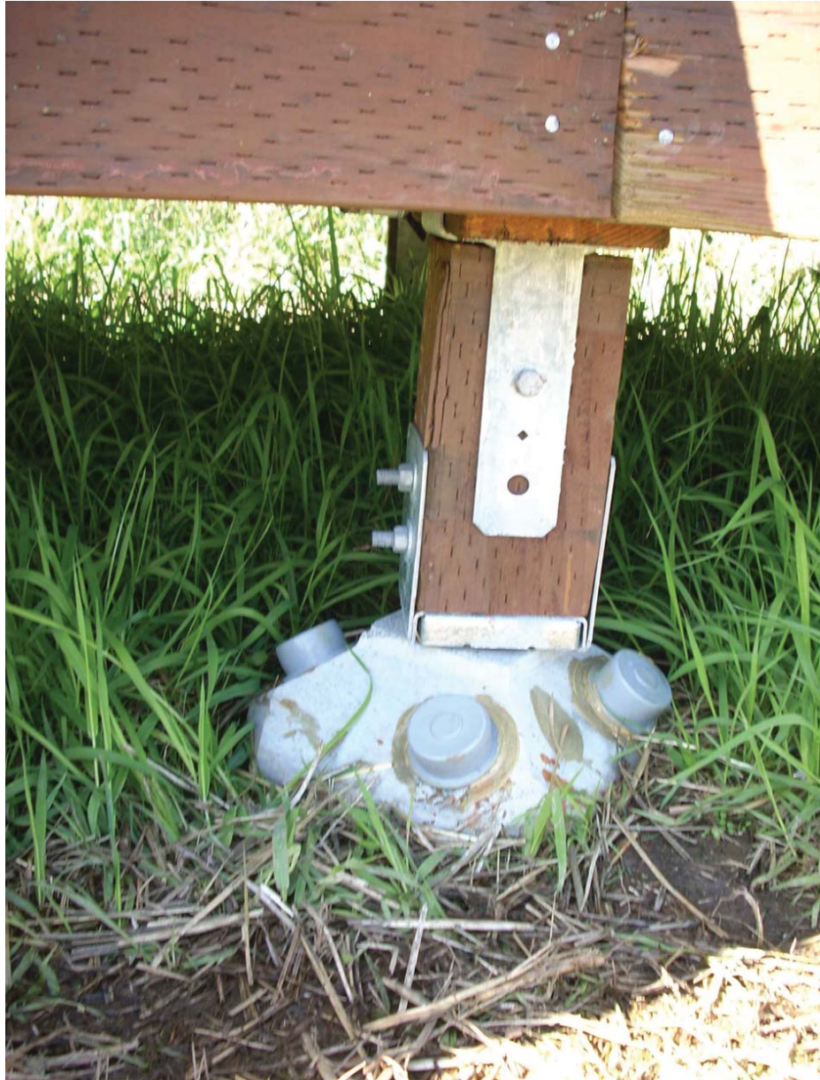
Figure 6.38: Pier-Type Minimal Excavation Foundation
