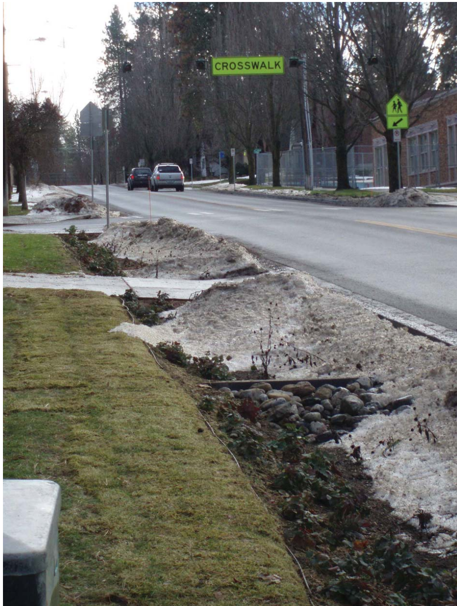
Figure 3.4: Bioretention Snow Storage
